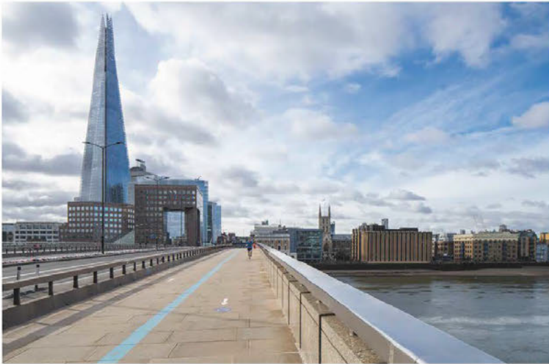
Existing view from north of London Bridge
