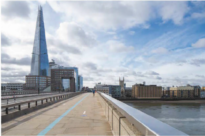
Existing view from north of London Bridge
